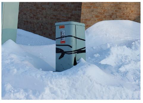
21. This photo from State Road, Hortonville, WI, shows two damaged splices wrapped in orange plastic coverings. Once the wrap deteriorates, wires are exposed to weather and animals. Damaged wires cause service outages.
