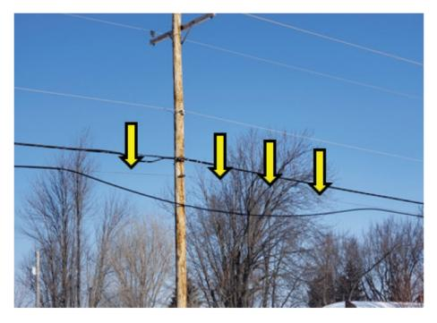
17. This photo from Green Bay Road, Neenah, WI, shows a double-pole. The old pole (right) has only AT&T equipment attached to it. AT&T has not moved its facilities to the new utility pole. As a result, AT&T's equipment remains connected to an old, deteriorating pole, causing potential service and safety concerns.
