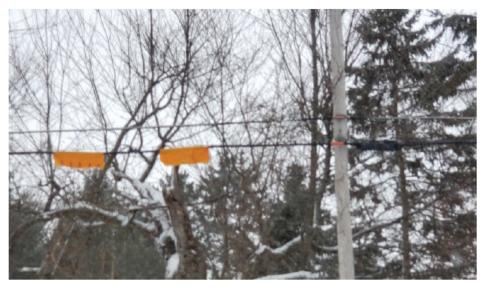
22. This photo from Breezewood Lane, Neenah, WI, shows unsecured cable. The cable should be secured to the utility pole. The wind blows the unsecured service cable, damaging the copper inside the wire and causing service issues. In addition, this cable is within reach of passersby, causing a public safety hazard.
