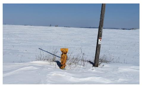
12. This photo from Clancy Road, Greenleaf, WI, shows an unsecured hanging terminal. The terminal should be secured to the utility pole. The terminal can fill with water, deteriorating wires and leading to service issues. In addition, a hanging terminal presents a public safety hazard.
