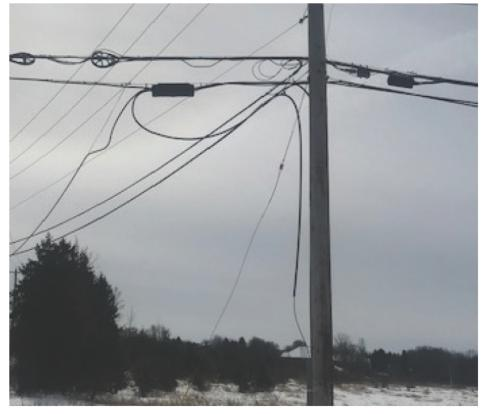
3. This photo from County Road, Neenah, WI, shows a severely damaged splice terminal. The terminal's protective case is hanging open, leaving wires exposed to weather and animals. Damaged wires cause service outages.
