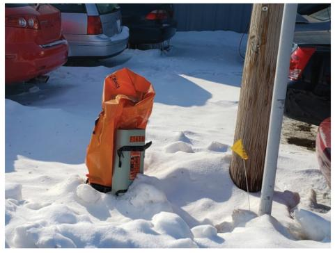
19. This photo from West Spencer Street, Appleton, WI, shows a rotting pole. AT&T's equipment is the only equipment that remains. AT&T has not moved its facilities to the new utility pole. As a result, AT&T's equipment remains connected to an old, deteriorating pole, causing potential service and safety concerns.
