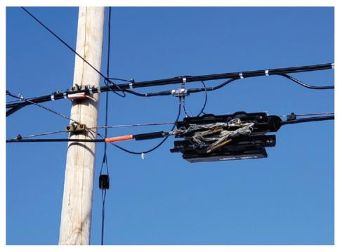
10. This photo from Rexford Road, Shiocton, WI, shows a damaged pedestal. Its protective cover is missing, replaced with a black plastic covering. This plastic covering will fall off or deteriorate over time, leaving wires exposed to weather and animals. Damaged wires cause service outages. In addition, the exposed wires are a public safety hazard.
