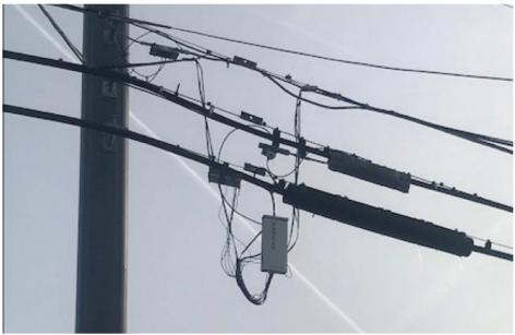
13. This photo from High Street, Wrightstown, WI, shows a double-pole. The old pole (left) has only AT&T equipment attached to it. AT&T has not moved its facilities to the new utility pole. As a result, AT&T's equipment remains connected to an old, deteriorating pole, potentially leading to service and safety concerns.
