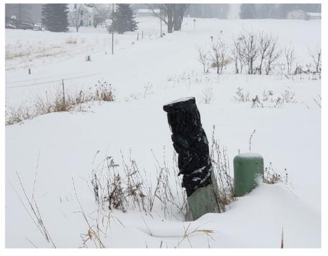
11. This photo from Clancy Road, Greenleaf, WI, shows a damaged pedestal. Its protective cover is missing, replaced with an orange plastic covering. This plastic covering will fall off or deteriorate over time, leaving wires exposed to weather and animals. Damaged wires cause service outages. In addition, the exposed wires are a public safety hazard.
