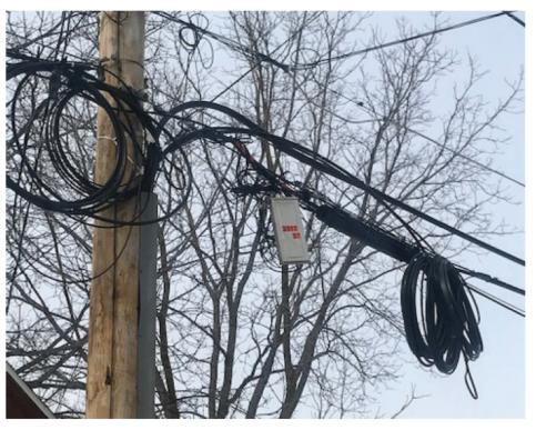
16. This photo from County Road, East Freedom, WI, shows an unsecured cable. The cable should be secured to the lash (yellow arrows) and the utility pole. The wind blows the unsecured cable, damaging the copper inside the wire, causing service issues, and straining the properly lashed cable.
