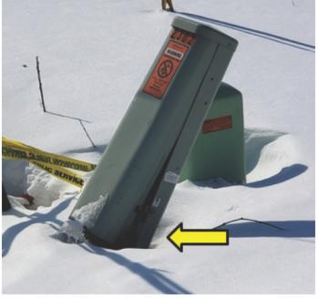
5. This photo from North Westhill Boulevard, Appleton, WI, shows a damaged pedestal. Its protective cover is missing, partially replaced with an orange plastic covering. This plastic covering will fall off or deteriorate over time, leaving wires exposed to weather and animals. Damaged wires cause service outages. In addition, the exposed wires are a public safety hazard.
