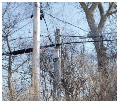
18. This photo from Plainview Drive, Oshkosh, WI, shows a damaged pedestal. Its protective cover is missing, replaced with an orange plastic covering. This plastic covering will fall off or deteriorate over time, leaving wires exposed to weather and animals. Damaged wires cause service outages. In addition, the exposed wires are a public safety hazard.
