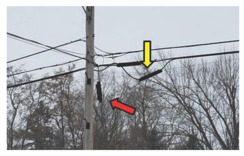
7. This photo from Spencer Street, Appleton, WI, shows unsecured cables. The cables are meant to be secured to the utility pole, not merely taped to the pole with electrical tape (yellow arrow), or secured to a lash (red arrow). The wind blows the unsecured service cable, damaging the copper inside the wire and causing service issues. In addition, this cable is within reach of passersby, causing a public safety hazard.
