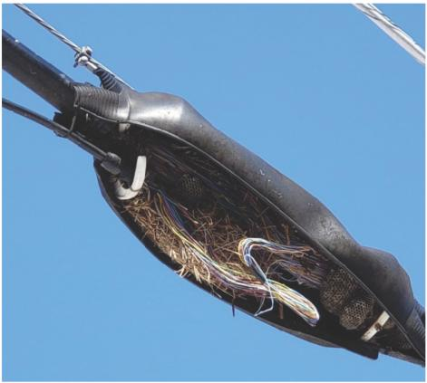
2. This photo from South Division Street, Port Washington, WI, shows unsecured cable. The cable should be secured to the utility pole. The wind blows the unsecured service cable, damaging the copper inside the wire and causing service issues. In addition, this cable is within reach of passersby, causing a public safety hazard.
