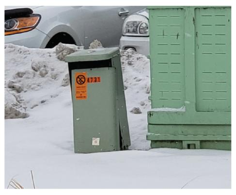
24. This photo from Greenville Drive, Greenville, WI, shows a damaged pedestal. Its protective cover is missing. Wires are exposed to damage from weather and animals. Damaged wires cause service outages. In addition, the exposed wires are a public safety hazard.
