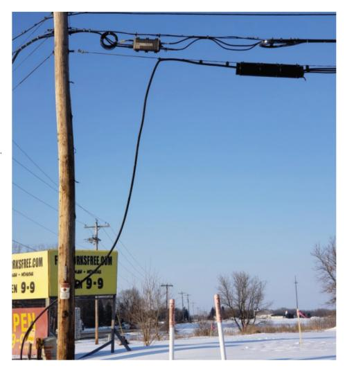
23. This photo from West Wisconsin Avenue, Appleton, WI, shows a damaged pedestal. Its protective cover is unsecured. Wires are exposed to damage from weather and animals. Damaged wires cause service outages. In addition, the exposed wires are a public safety hazard.
