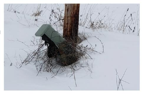
9. This photo from County Road, East Freedom, WI, shows a severely damaged splice case. The splice's protective case is hanging open, leaving wires exposed to weather and animals. Damaged wires cause service outages.
